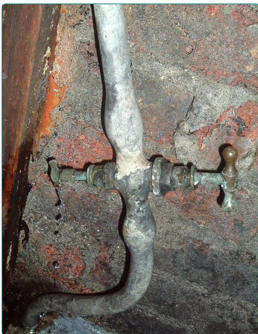
Figure 5 – Example lead pipe arrangement
