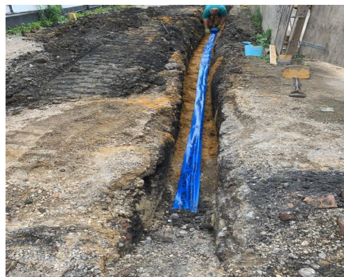
Example above showing depth markers and below showing new water pipes with sand backfill and water marker tape.
