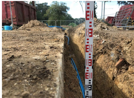
Example above showing depth markers and below showing new water pipes with sand backfill and water marker tape.
